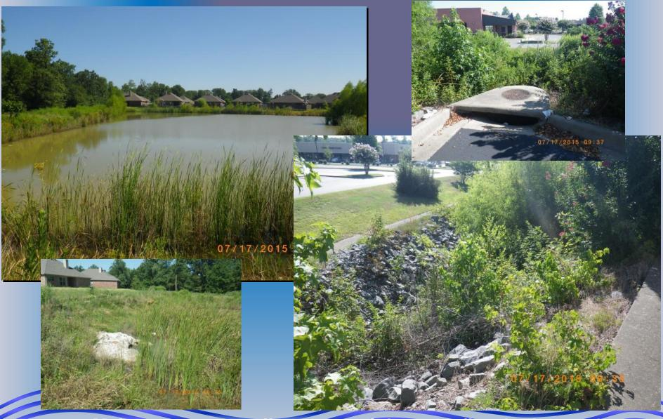
Main purpose usually to control the peak flow hydrograph
