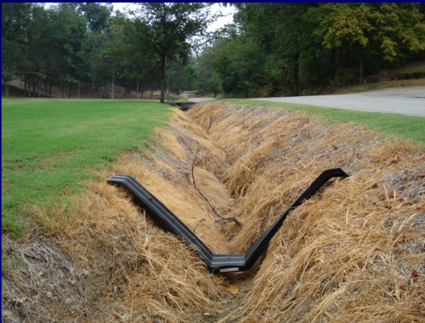
2' ditch, Dogwood Lane
