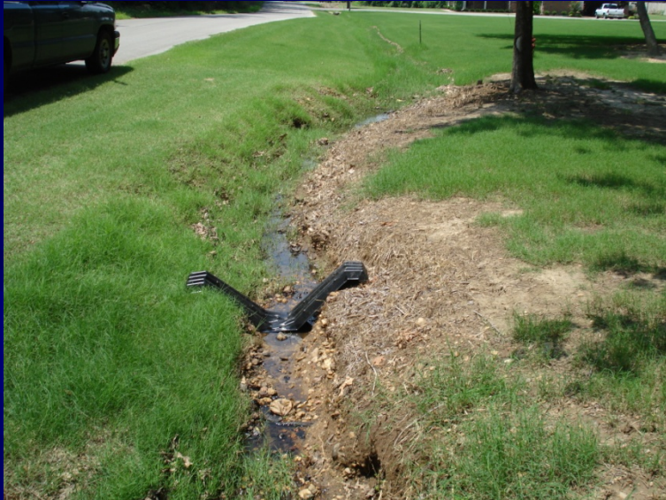
12" HDPE for portions
