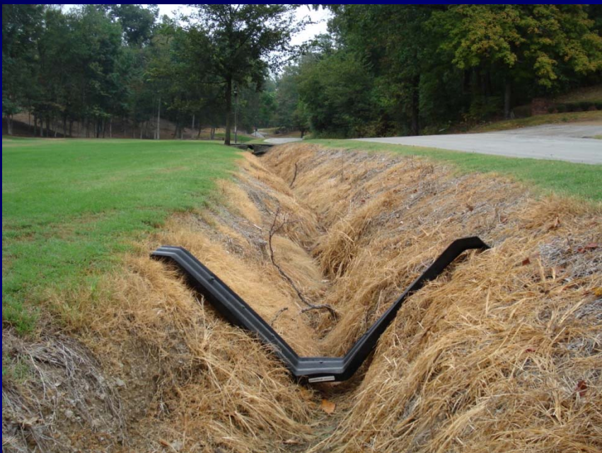
2' ditch, Dogwood Lane
