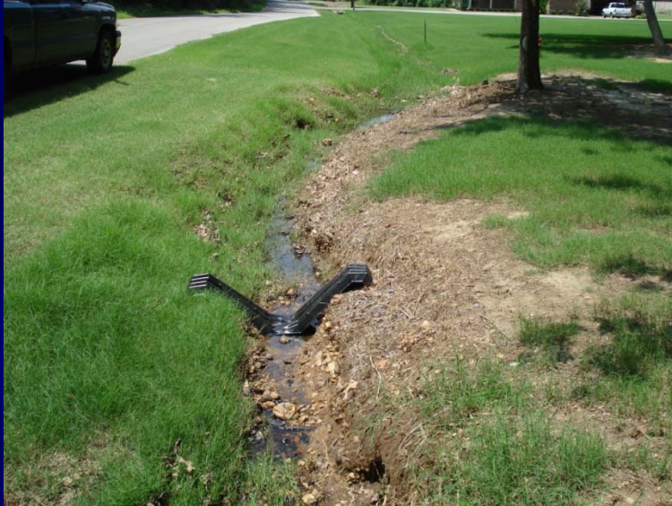
12" HDPE for portions
